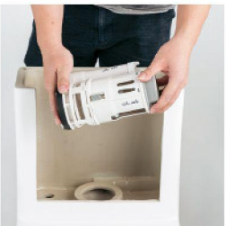
Install the water flush valve
