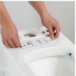
Aim the slot at the hole in the toilet cover
