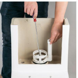
Tighten the water outlet valve base screw
