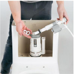
Unscrew the water inlet valve screw
