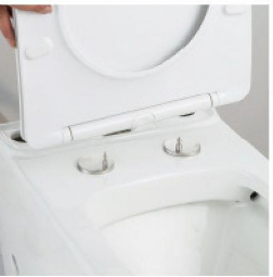
Install the screws from both sides
