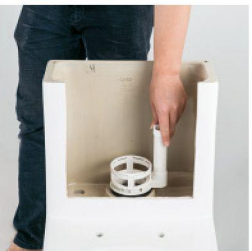
Tilt into the water outlet valve base
