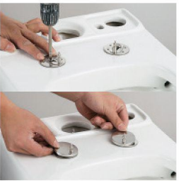
Install the screws from both sides
